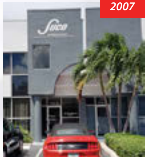
SUCO Technologies Boca Raton, USA
