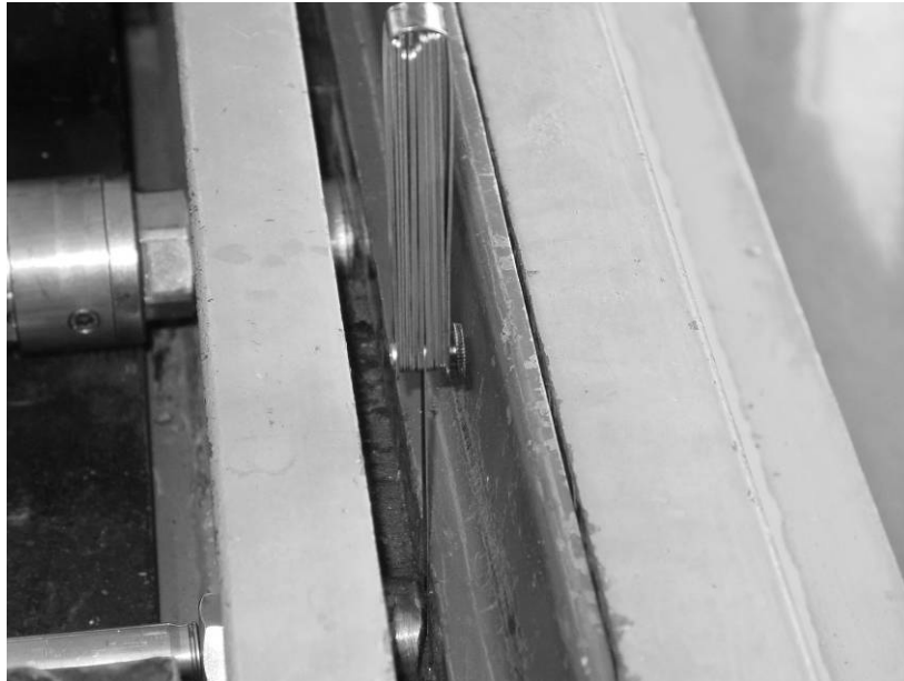
Fig. 111: Measure gap between tongue detector block and point tongue
