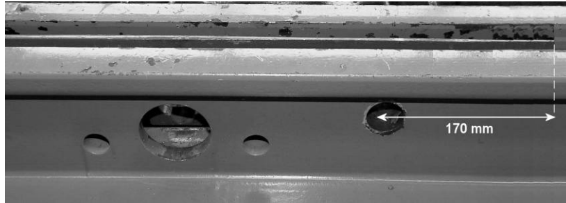
Fig. 34: Clearance between the gap for the detector rods and the tip of the switch tongue
