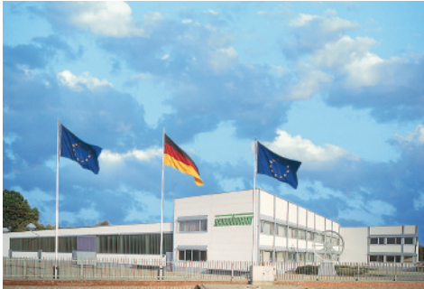
Production plant in Neuenhaus
