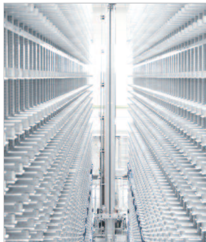
254 Regalbediengeräte Storage and Retrieval systems
