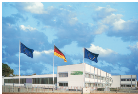
Production plant in Neuenhaus
