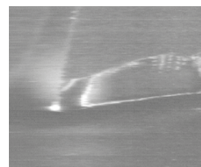
Defect example: missing coating
