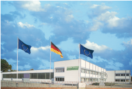
Production plant in Neuenhaus
