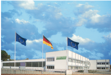
Production plant in Neuenhaus
